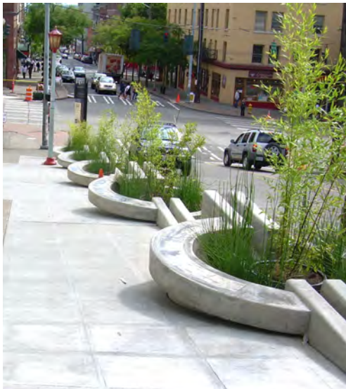
Cascading stormwater feature: These cascading concrete pools and landscaping along Maynard in the International District are a good example of capturing and controlling the flow of stormwater on a sloping site in an artistic and engaging design.
