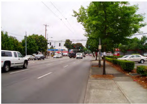
Most of the existing sidewalks along Rainier Ave. are narrow and provide no buffer from the passing car traffic for pedestrians.
