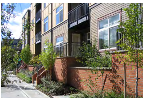
Ground-level entries: The setback entrance to an individual residential unit clearly marks the entry, and provides usable private outdoor space that successfully transitions a resident or visitor from the public to the private realm.
