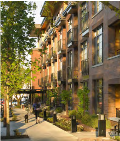
Finely scaled building features & rhythm: This building increases the level of detail below 30 feet in height, using operable windows with divided panes, natural and durable materials, and pedestrian lighting. Window headers are expressed with brick soldier courses. (Ankrom Moisan Architects)
