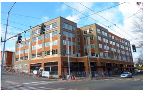
The Claremont Apartments accentuates the corner of Rainier Ave. and S. Walden St. with a prominent entry, setbacks, and building form.
