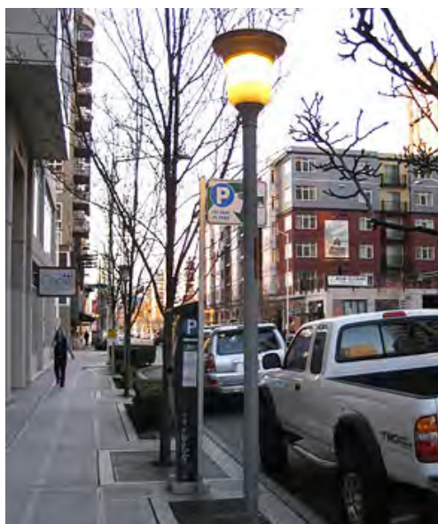
Pedestrian lighting: Pedestrian-scale lighting creates a more intimate streetscape while providing safety benefits beyond conventional “cobrahead” lights. All luminaires should have a cutoff above the lightsource, directing light down and away from living quarters.
