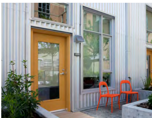
High quality windows: Aluminum windows integrate nicely with the metal facade on this residential building. (Gregg Galbraith Photography)
