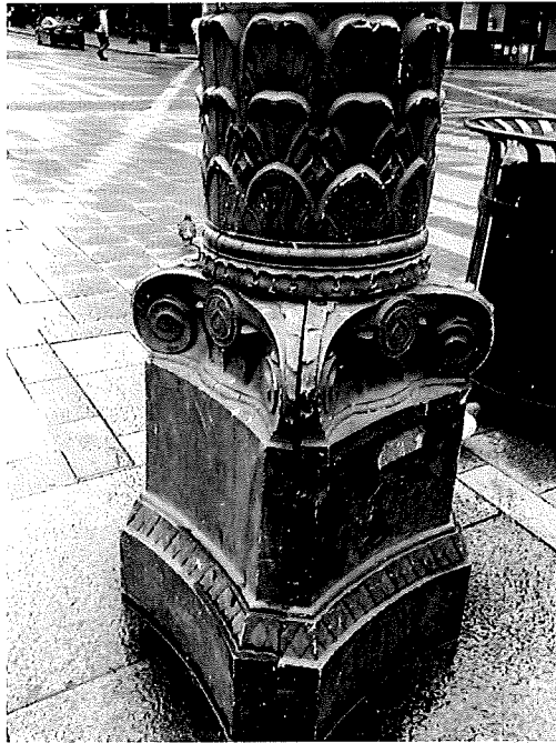
Light base is cracked. Some electrical boxes do not seem to be working, small amount of graffiti.
