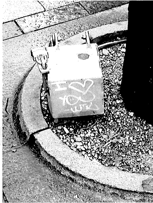
Light base is cracked. Some electrical boxes do not seem to be working, small amount of graffiti.
