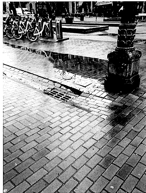
Cracked Pavers at the north entryway off of South Washington Street.
