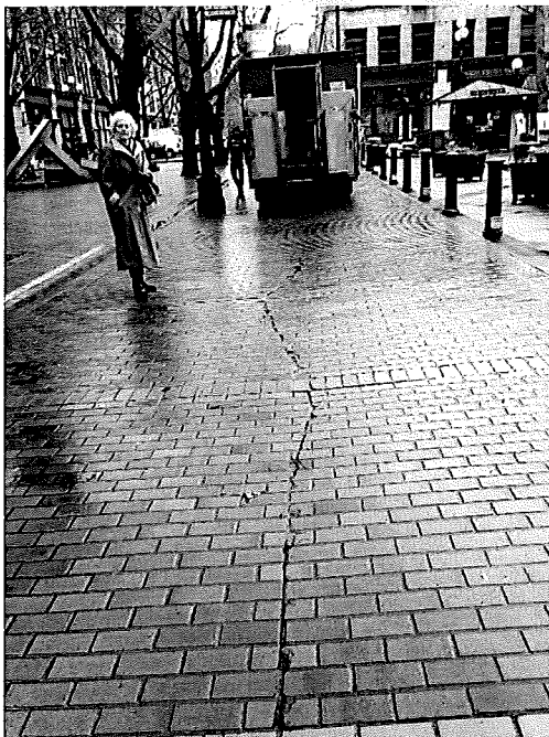
Cracked pavers the entire length of Occidental Ave South.
