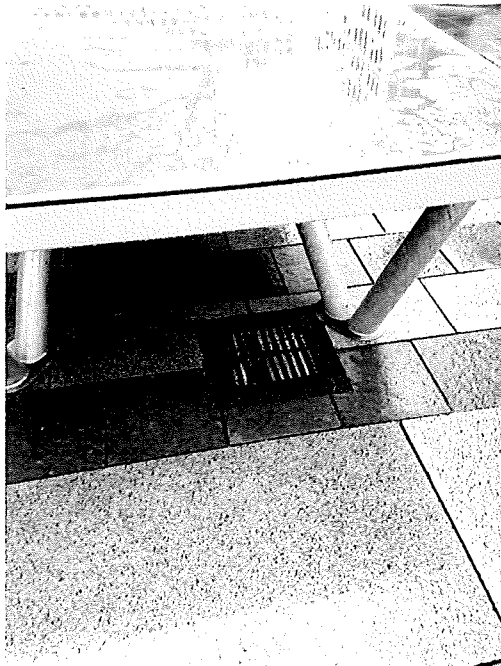
Light base is cracked. Some electrical boxes do not seem to be working, small amount of graffiti.
