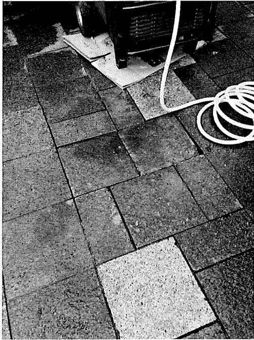
Pavers are loose and broken from truck access traffic off of Pine Street. Food trucks need to be using oil pans while parked.
