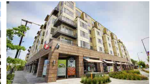
3- STATION AT OTHELLO PARK APTS. 4219 S OTHELLO ST | APARTMENT Facade is flush with the street/sidewalks allowing for space in the back for a residential courtyard. By setting the front facade against the sidewalk the retail and residential entries are more defined resulting in a positive use of the site.
