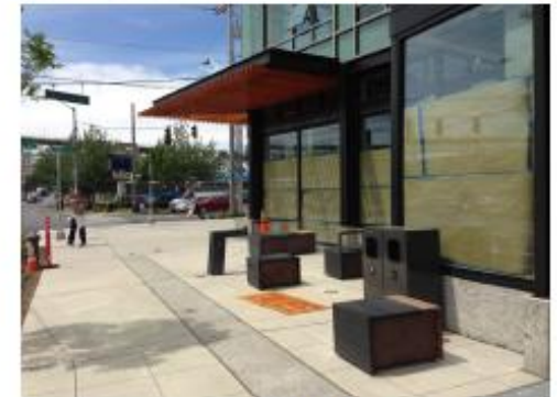
A small setback can be used to create room for customer amenities like bicycle parking, seating, or lean rails close to bus and rail stops.
