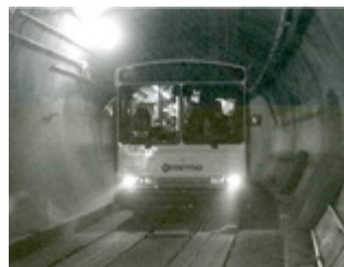
▲ Metro bus in tunnel. Circa 1980s-1990s Credit: King County Office of Information Resource Management Printing and Graphic Arts photographs. Series 1147, Box 1, Folder 27.
