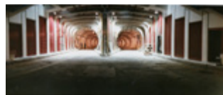
▲ Third Avenue tunnel entrance at University Street Station. April 1990 Credit: King County Office of Information Resource Management Printing and Graphic Arts photographs. Series 1147, Box 1, Folder 25.
