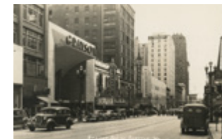
▲ The Capitol Theatre, once part of the Telenews circuit, on Third Avenue facing south from Pine Street. Circa 1942 Credit: Seattle Public Library
