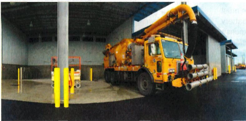
South Service Center treatment facility
