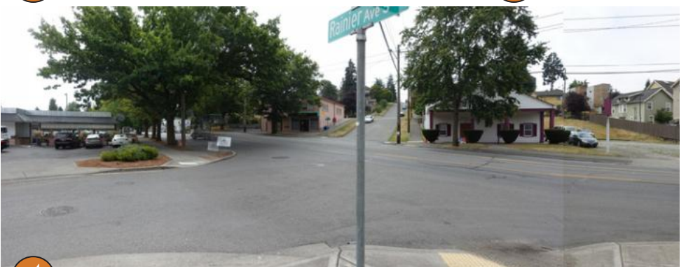
4 looking south at intersection of Rainier Ave S and 42nd Ave S
