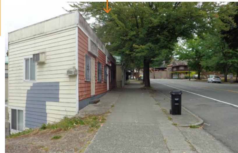
Sidewalk along Rainier Ave S
