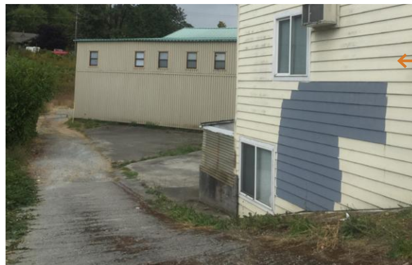
Bird's Eye View- looking northeast- Discontinuous alley/ does not continue directly eastward to 42nd Ave S
