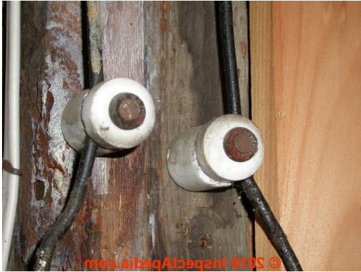
“knob and tube” wiring
