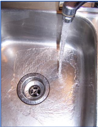
Toilets, Sinks, Showers, Washing Machines
