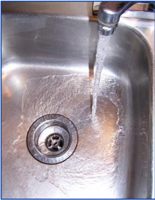
Toilets, Sinks, Showers, Washing Machines
