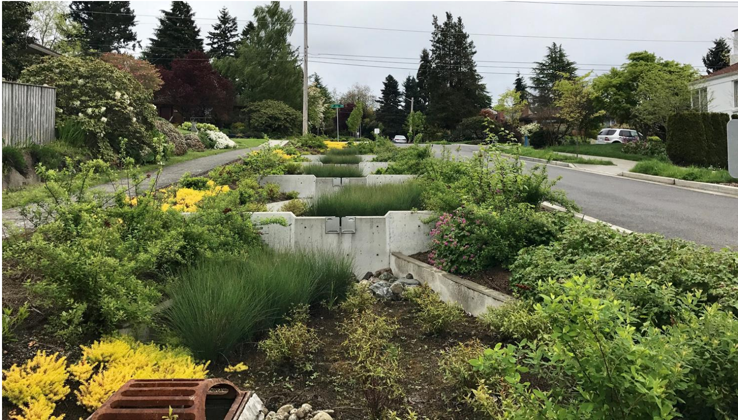
Green Stormwater Infrastructure: Venema Natural Drainage System
