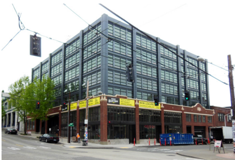
A successful example of an addition that was set back less than 15'. The contrast between the character structure and the new addition was achieved through materials, subdued colors, simple fenestration and changing the original vertical grid orientation to a horizontal emphasis.
