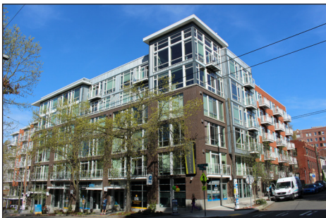
The storefronts on different levels accentuate the differences between the two building façades and appear to “step up” with the topography.
