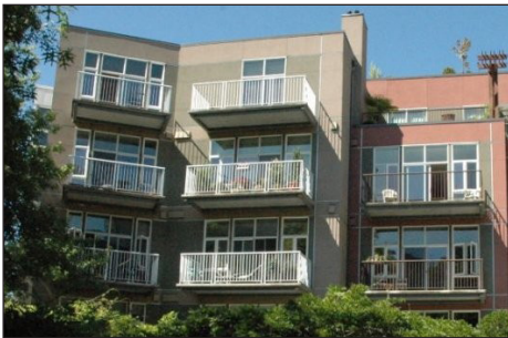
Usable balconies provide visual relief in addition to private open space. In this example, the balconies face the rear of the lot.
