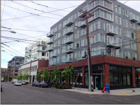
Large development site with massing that creates the appearance of a grouping of smaller structures.
