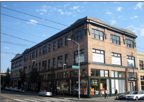
Ground level with tall floor-to-ceiling heights and high degree of transparency. Transparent windows and retail modules with individual entrances lend to human-scaled streetscapes.
