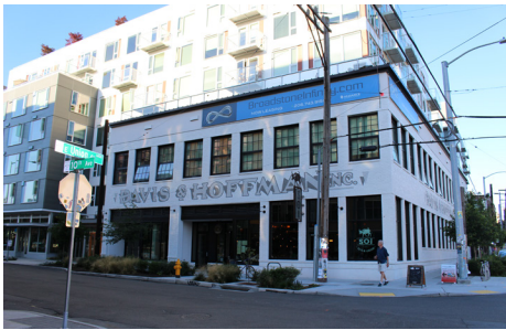
Examples of design approach using setbacks to distinguish character structures from new development.
