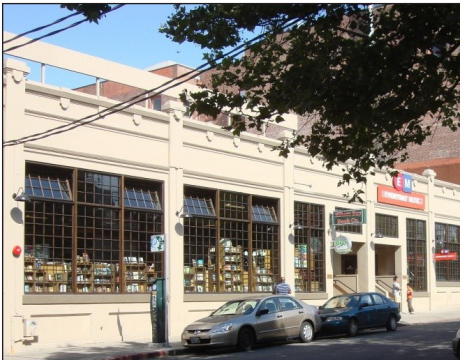
Renovated character structures that have retained character-defining elements.
