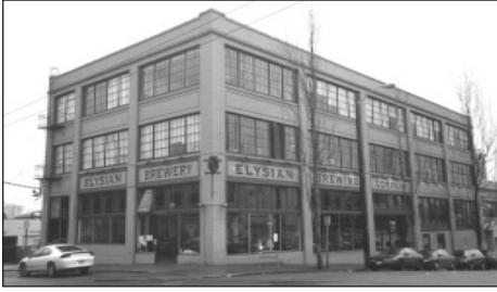
Elysian Brewery. Context—light industrial signage and building design; tall windows.
