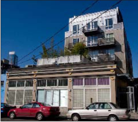
This addition is placed to the rear of the character structure and set well back from the street front, retaining the original proportions, scale and character of the main facade.
