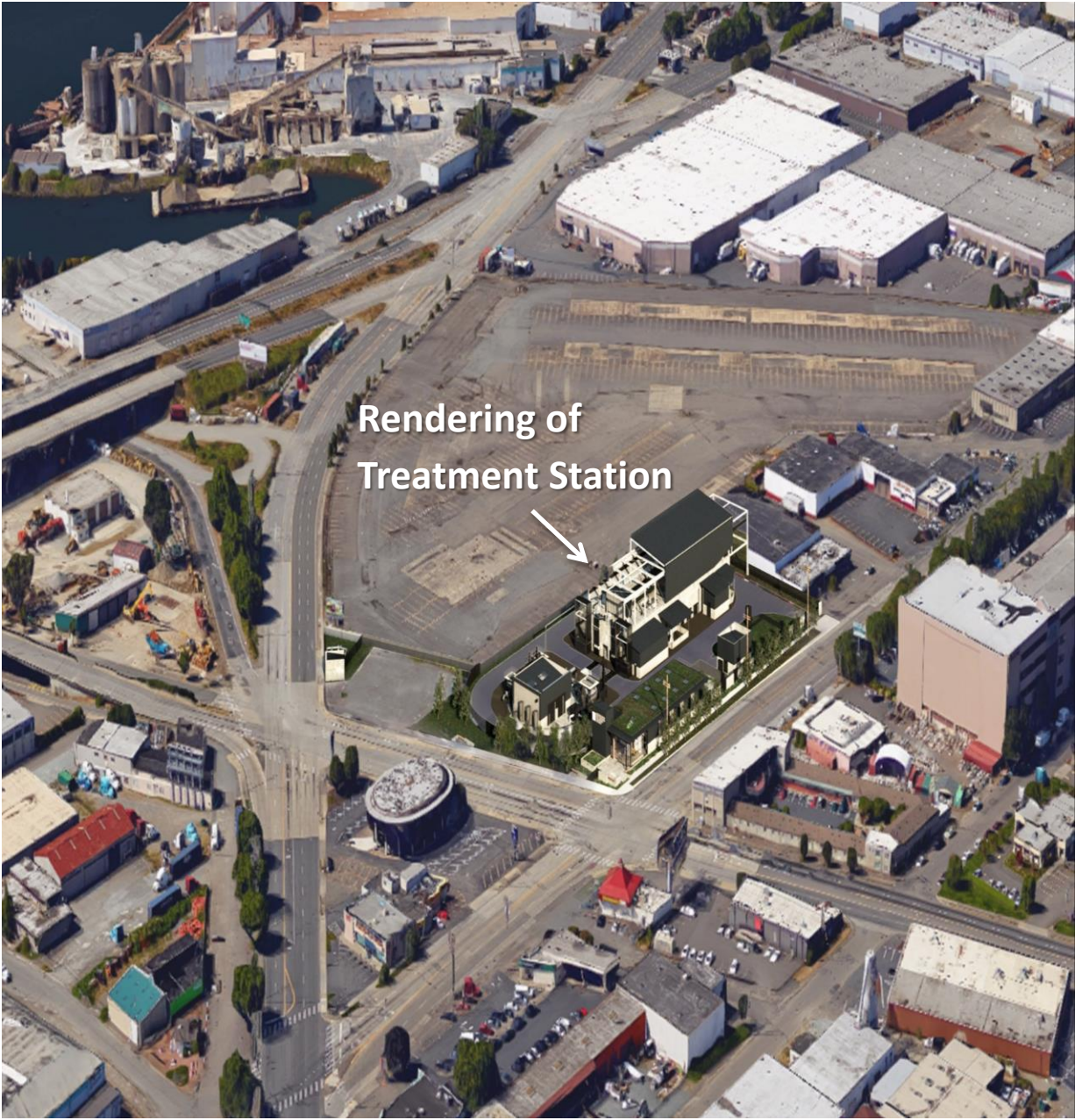
Attachment B: Rendering of the Georgetown Wet Weather Treatment Station, looking from the southeast
