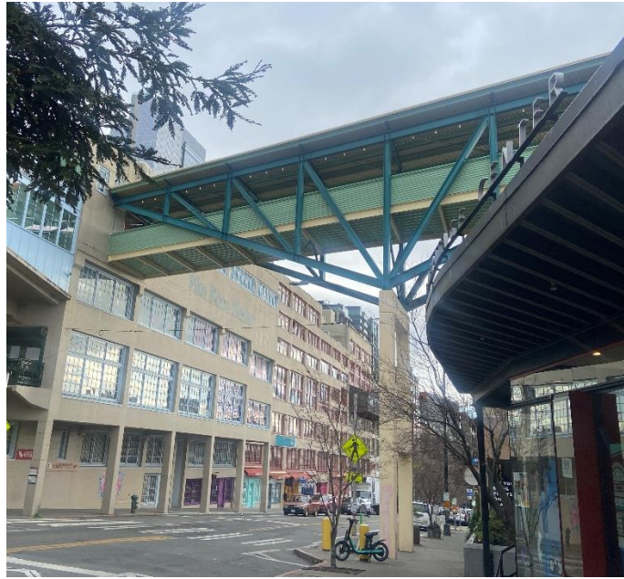
From Western Ave
