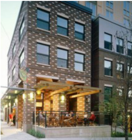
Durable materials at ground level.
