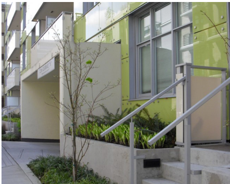
Conceal all underground parking from street views. Planting, artwork, or other uses can effectively screen parking.
