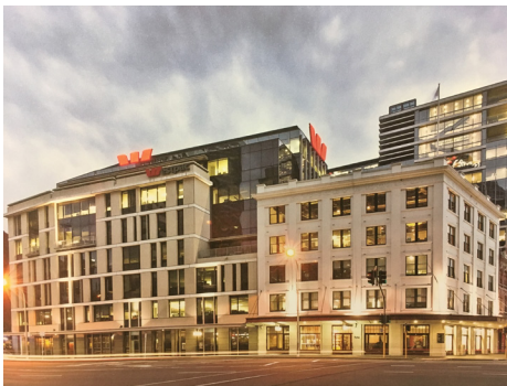
New (left) compatible with restored (right). Taller Portions stepped well back. The Britomart, Auckland, NZ.
