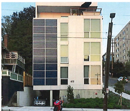
Solar panels add interest to this facade and help meet the building's energy needs.
