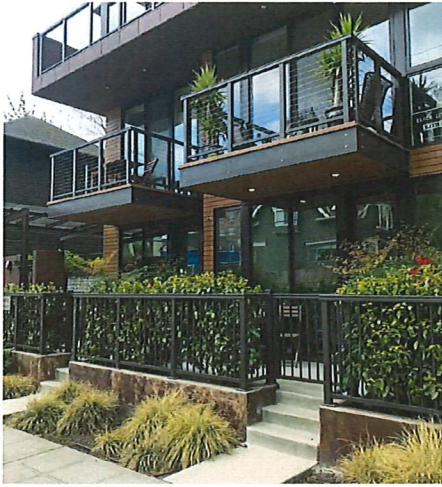
Low-level planting and fencing with a minor elevation change provides separation and security for ground-level housing along a busy street-edge. Upper level balconies are large enough for small groups and encourage social interaction.
