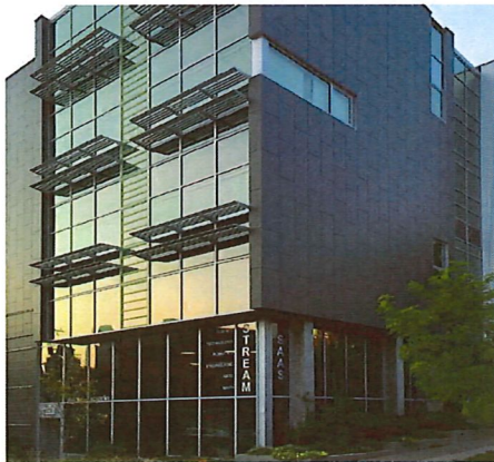
Sun shades reduce solar gain and cooling needs.
