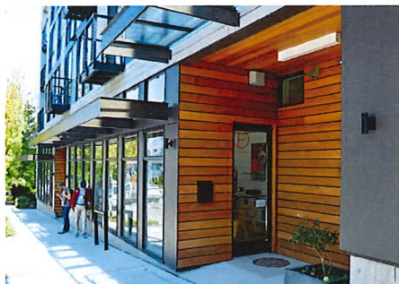
Street level facades step down to respond to local topography.
