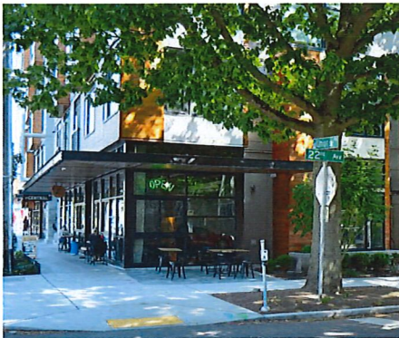
Development located on a corner site is designed to have an active retail edge and a quieter residential edge.
