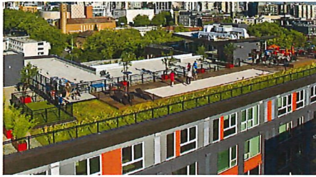
Green roofs provide habitat and reduce the heat island effect.
