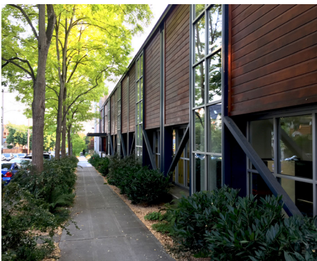
Choice and placement of materials create scale and texture for this school building.
