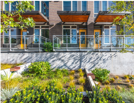
This system for reusing rainwater is attractive and functional.
