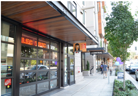
A well designed overhead weather protection is functional, attractive, and leaves adequate room for street trees.
