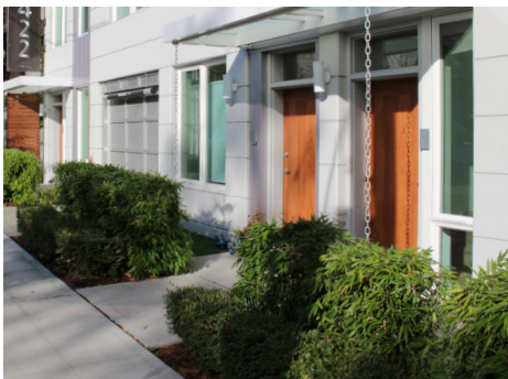
Translucent canopies and a mix of planting and hardscape help define the public to private transition for street facing apartments within a modest setback area.
