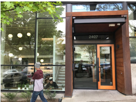
This north-facing live/work unit uses a high level of transparency to enliven the street edge, maximize daylight penetration, and connect the indoor and outdoor environments.
