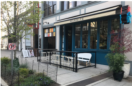
Small scale retail facade fits into the overall building concept and allows for personalization with color, signage and retractable canopy.
