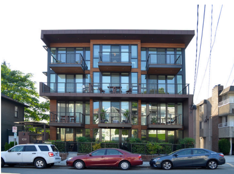
Wood planking is used to highlight the building's simple structure and balanced proportions.
