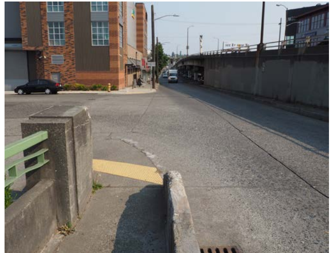
Ballard Bridge on-ramp at NW Ballard Way, looking north.
