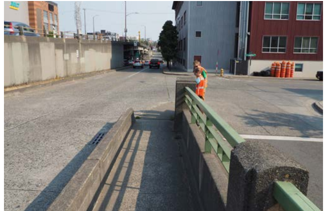
Ballard Bridge off-ramp at NW Ballard Way, looking north.
