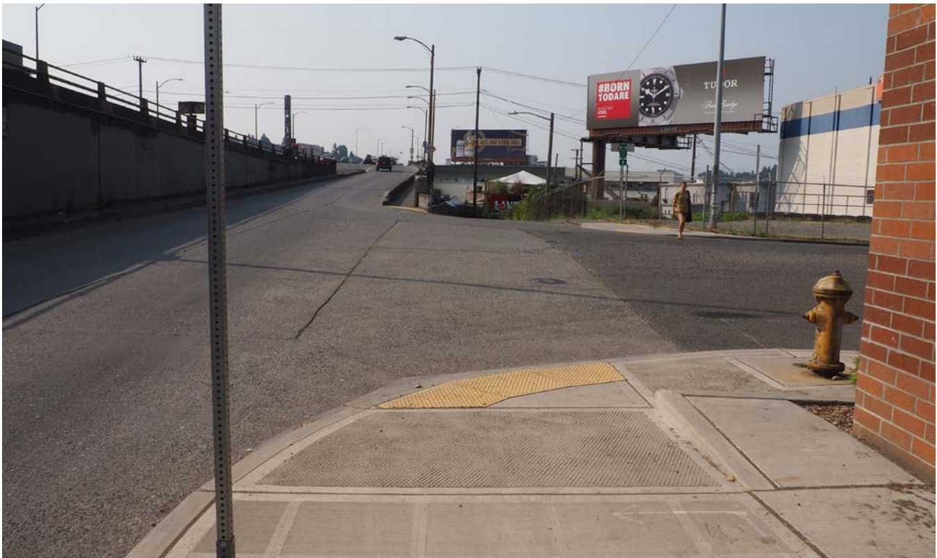
Ballard Bridge On-Ramp at NW Ballard Way, looking south.
