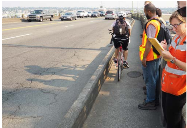
Ballard Bridge sidewalk, looking north.
