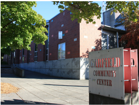
Garfield Community Center
