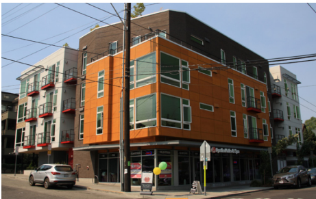
Articulated building massing both horizontally and vertically breaks down the building's scale.
