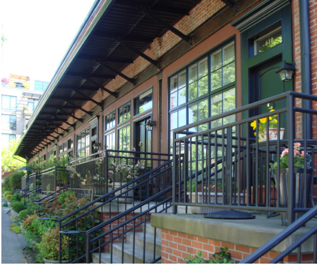
Raised entries that create a private stoop at residential entrances, with high transparency railings that facilitate street interaction.
