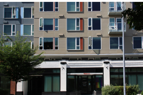
Preservation of the ground floor facade, with a compatible addition above retains a portion of the neighborhood's history.
