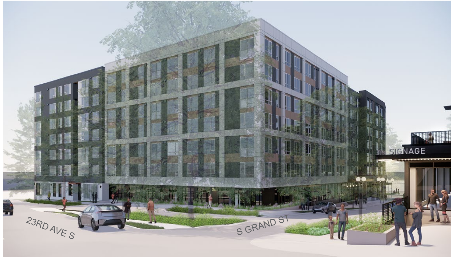
VIEW OF THE NORTH EAST CORNER OF THE SOUTH BLOCK FROM 23RD AVE S
