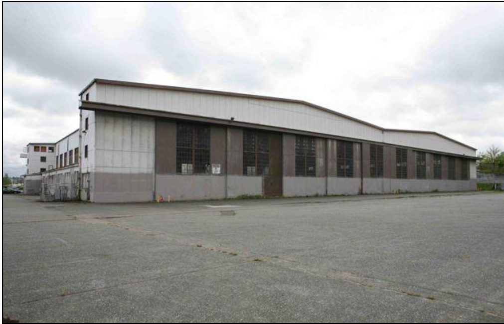
West Facade (Current construction condition)
