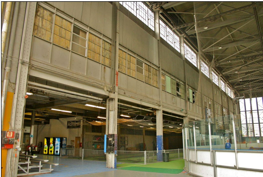
Photo by Megan Espinoza, 2010. Central Multi-Story Hangar Interior: Hangar Doors
