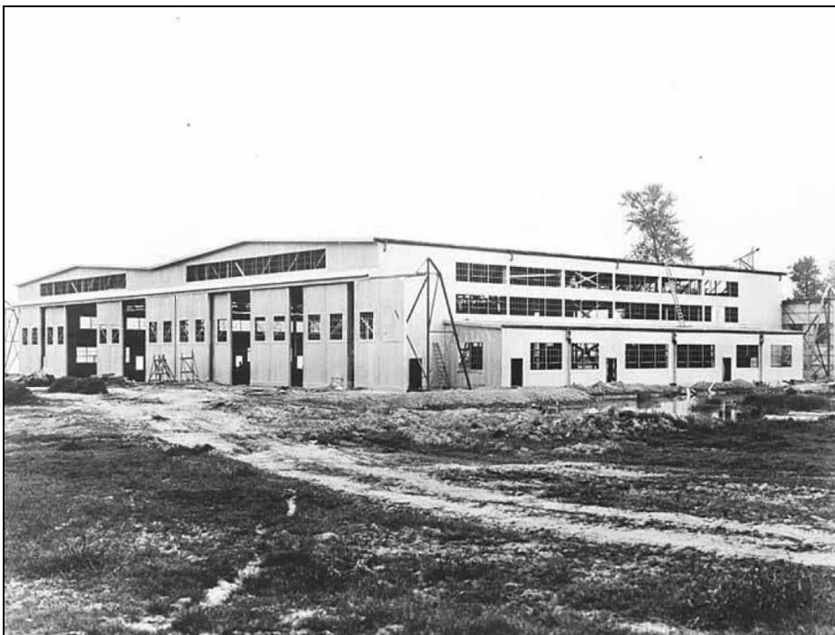
Completed land plane hangar. Photo Source: University of Washington Special Collections, Image No. SEA2804.
