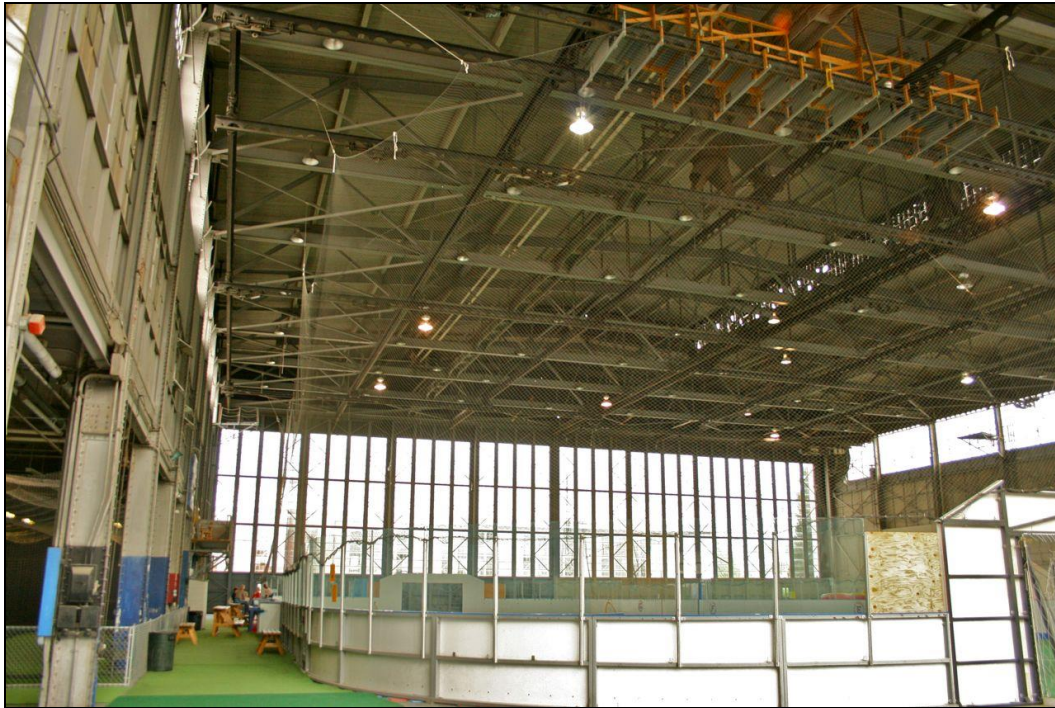
Photo by Megan Espinoza, 2010. Central Multi-Story Hangar Interior (Looking towards former shooting range that separates the large and small hangars.)
