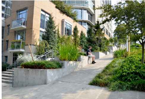
Accessibility of a sloping sidewalk is enhanced by resting spots and stair with handrails.
