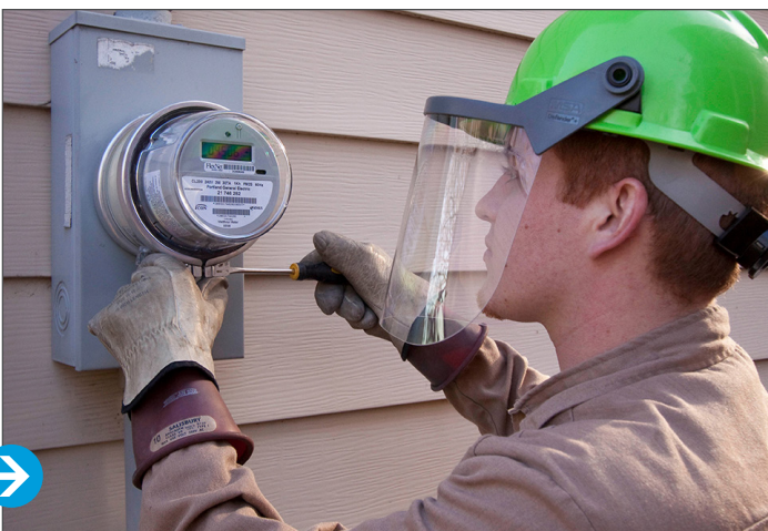
Smart meters enable two-way communication between energy user and utility, which helps the utility pinpoint inefficiencies and read energy usage remotely, reducing utility vehicle miles. (Posted to Flickr by Portland General Electric. Cropped. Creative Commons 2.0 Generic License (CC BY 2.0) https://creativecommons.org/licenses/by/2.0/legalcode .)
