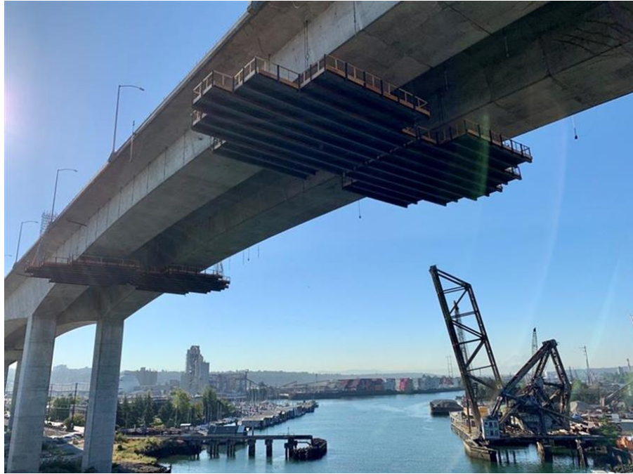
Work platforms installed in July
