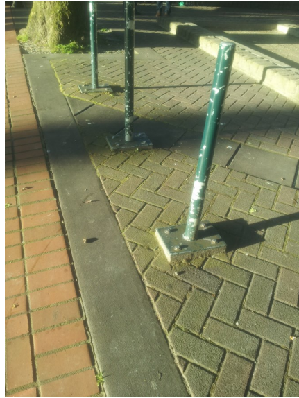
Bench fence post - chipped and need to be painted.
