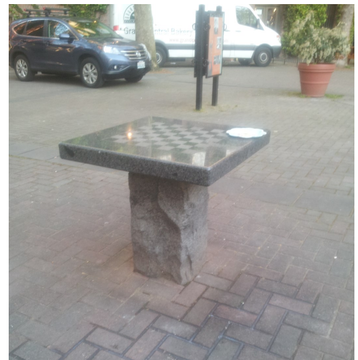
Chess tables - chipped on edges and graffiti
