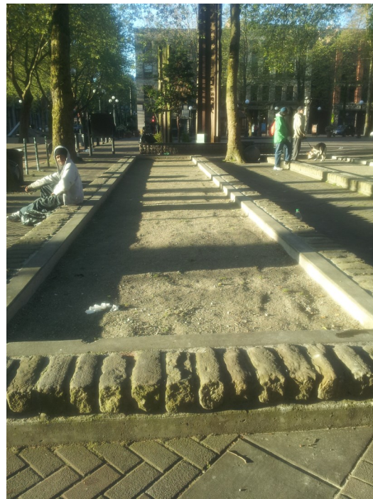
Bocce courts—surface needs to be redone. Pavers around the edge of the courts are chipped and damaged.
