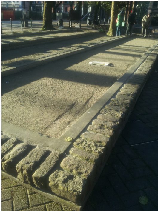
Bocce courts—surface needs to be redone. Pavers around the edge of the courts are chipped and damaged.
