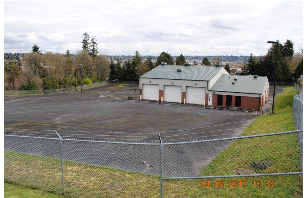
OMS 245 / Maintenance Shop (8,100 sq. ft.)
