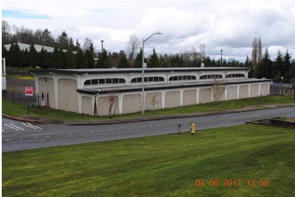
AMSA 222 / Maintenance Shop (6,400 sq. ft.)
