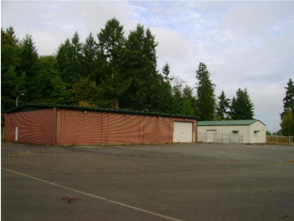
Building 211 / Unheated Storage (6,000 sq. ft.)
