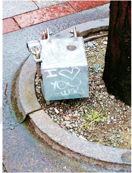
Light base is cracked. Some electrical boxes do not seem to be working, small amount of graffiti.
