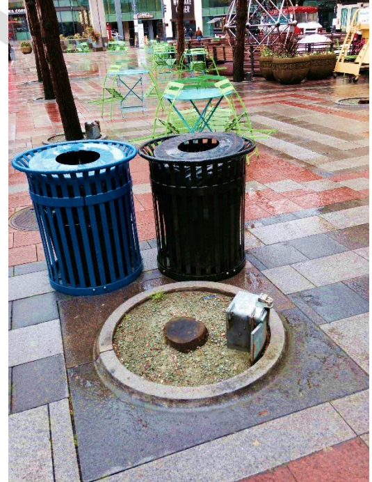
SPR signs need improvement. Two trees are missing from the center of the park.
