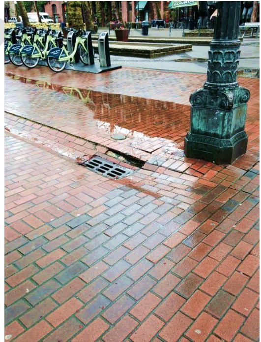
Cracked Pavers at the north entryway off of South Washington Street.
