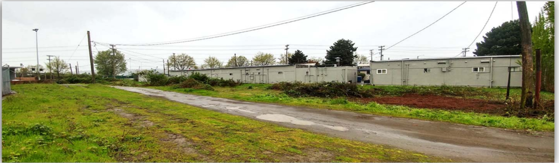
Figure 16. View of the flume property from South Myrtle Street
