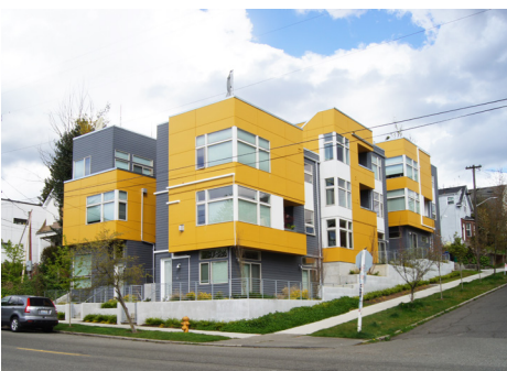
Broken-up building massing avoids a monolithic form.
