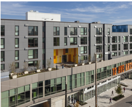
Upper floor setback creates a usable outdoor "community porch" space.
