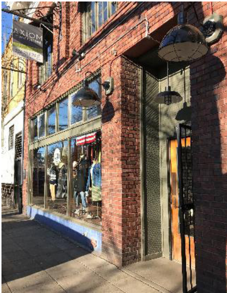
At the street level, a variety of textures such as blade sign, uneven brick, pendant lights, and windows add texture and scale that is perceptible at a walking pace.
