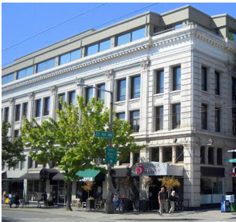
This strong facade composition, detailing, and high-quality materials establish a clear commercial character.
