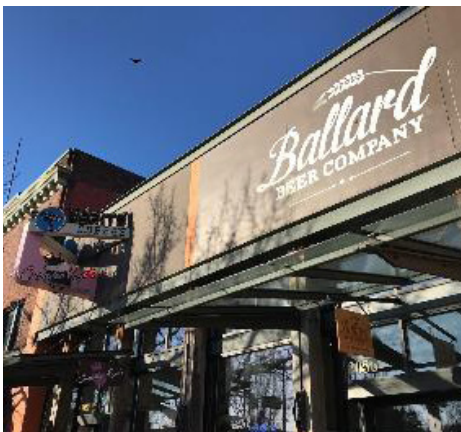
The variety of signs are integrated with the building architecture.
