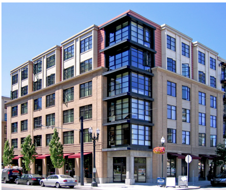
The vertical and horizontal banding is expressed differently in the lower and upper portions of this building, providing a unifying theme while reducing the perceived bulk.
