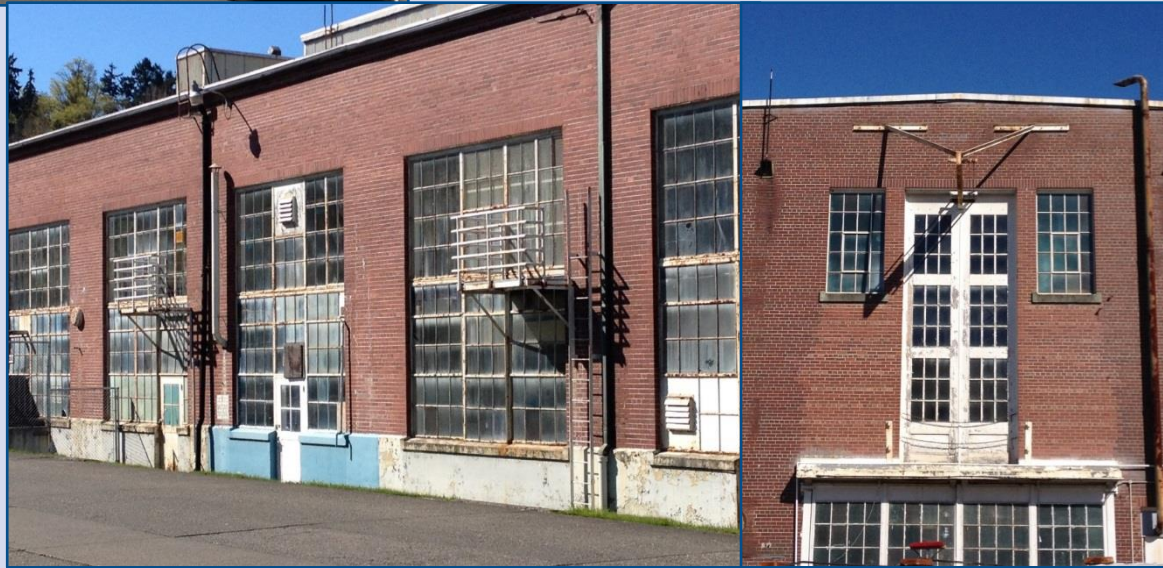
BUILDING 2 ASSEMBLY/REPAIR SHOP (1929 W/ ADDITION 1939-1944)
