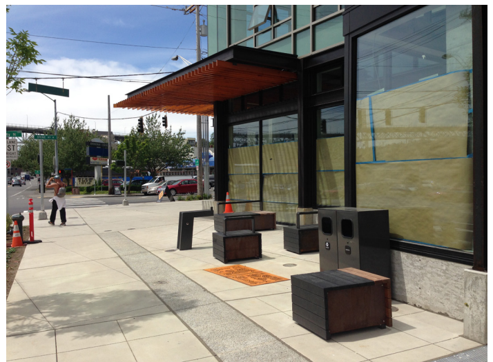
A small setback can be used to create room for customer amenities like bicycle parking, seating, or lean rails close to bus and rail stops.
