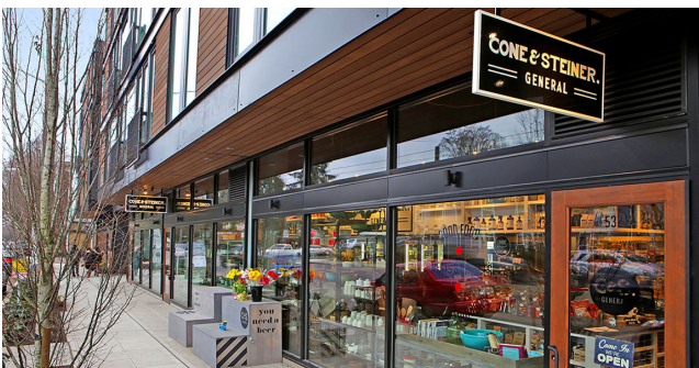
A small setback can be used for outdoor displays where sidewalk widths are limited or where pedestrian volumes are high.
