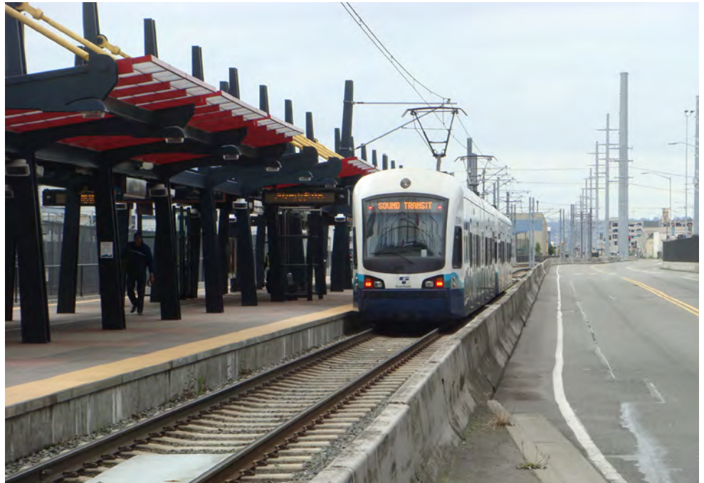
A light rail train approaches the Stadium LINK station.
