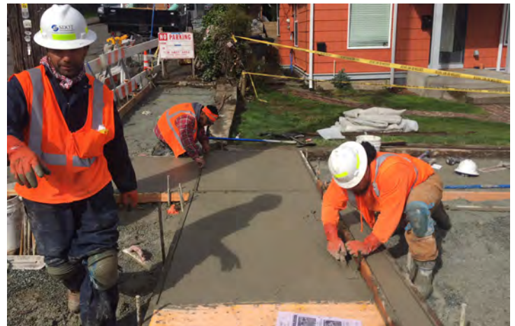
SDOT crew members replace a traditional sidewalk in Seattle.
