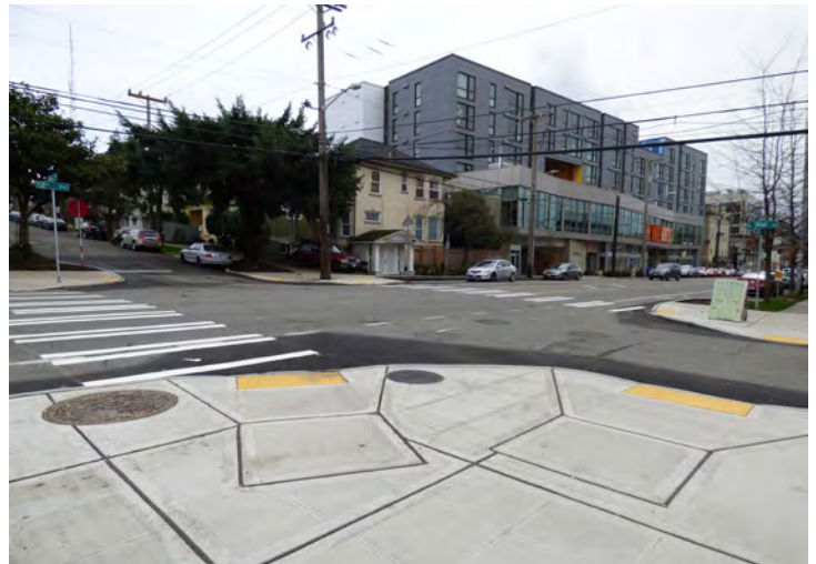
Newly constructed curb ramp and crossing improvement.
