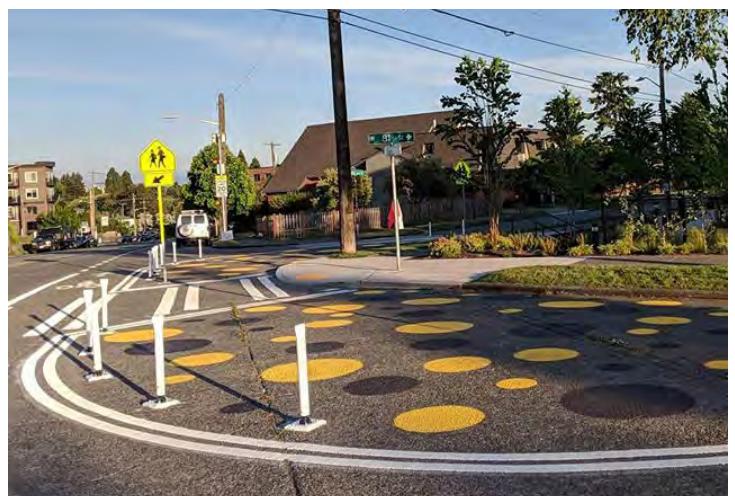
Low-cost crossing improvement that provides a barrier between people walking and people driving.
