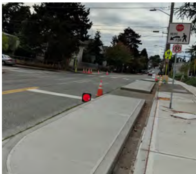
Newly constructed curb ramp and crossing improvement.
