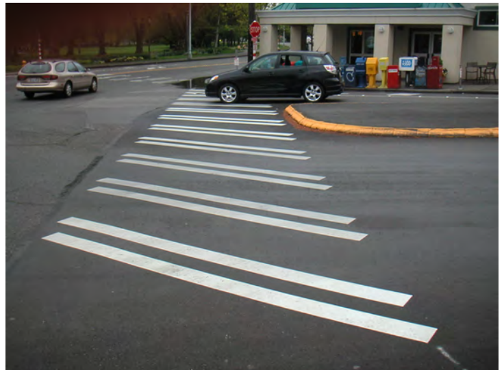
Crosswalk repainting (after).
