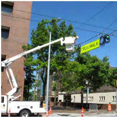
SDOT crew member installs a crosswalk sign in the Capitol Hill neighborhood of Seattle.
