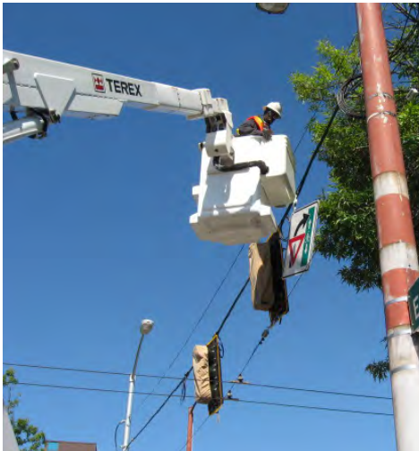
Crew member improving a traffic signal in Seattle's Capitol Hill neighborhood.
