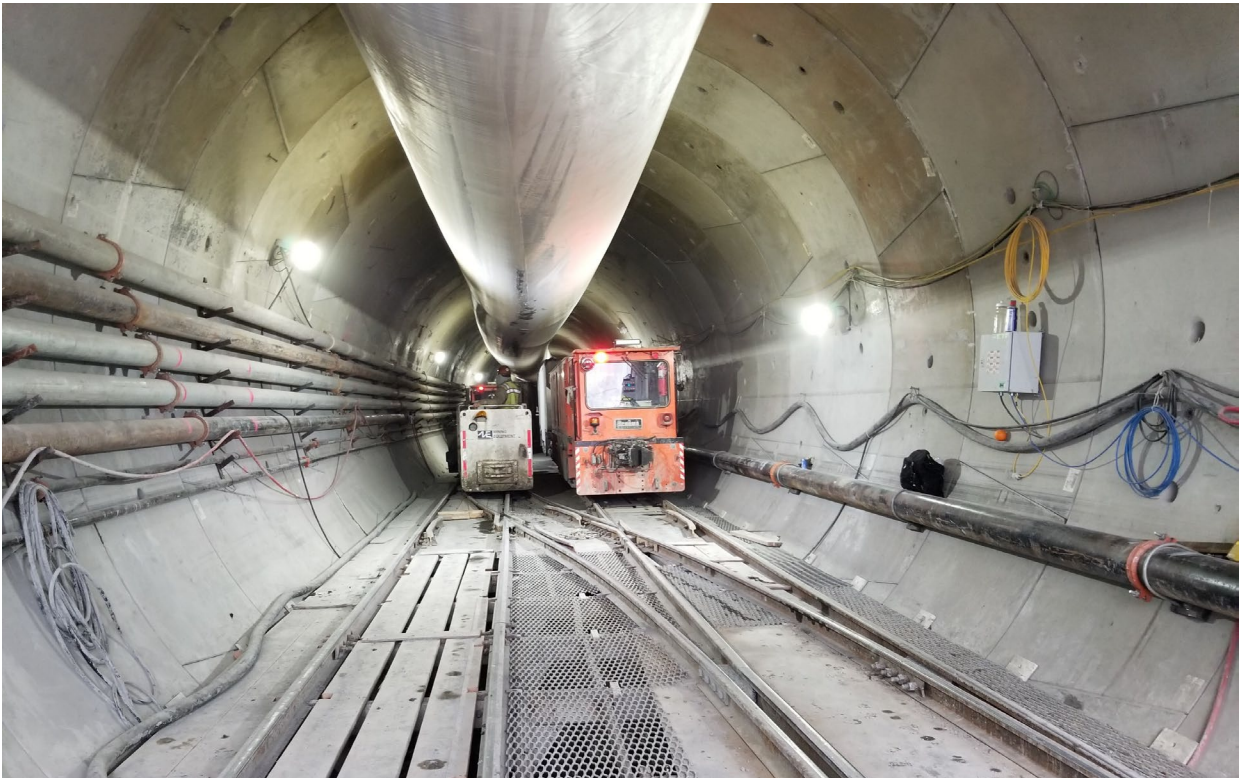
Ship Canal Water Quality Project – under construction
