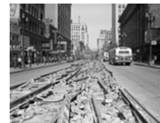
▲ Removal of the tracks on Third Avenue near University Street. June 8, 1943 Credit: Seattle Municipal Archives
