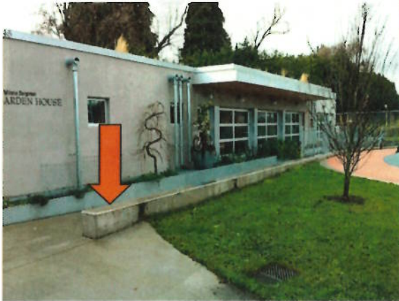
“Tuning fork” frame will sit atop concrete wall, with descending heights to meet existing fence height at far end.
