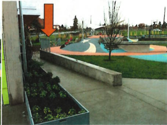
“Tuning fork” frame will sit atop concrete wall, with descending heights to meet existing fence height at far end.
