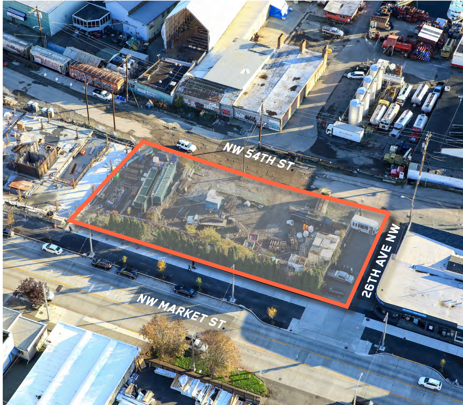
Aerial View Looking Southeast
