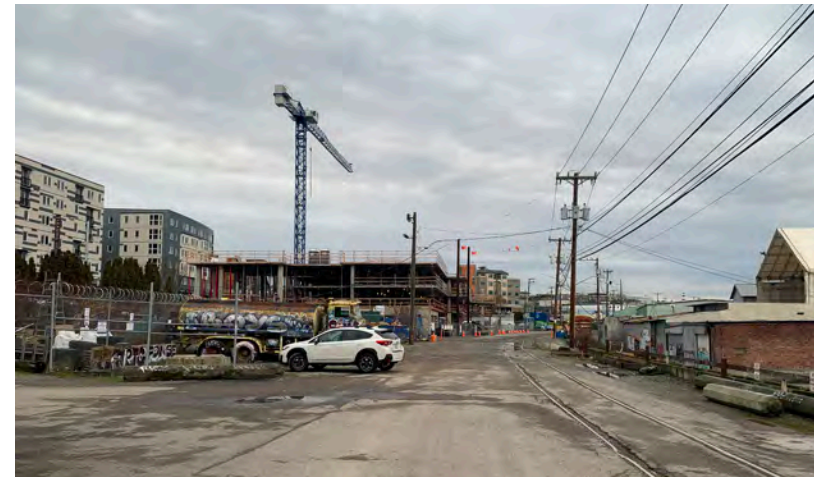
9. SOUTH EDGE OF PROPERTY LOOKING EAST
