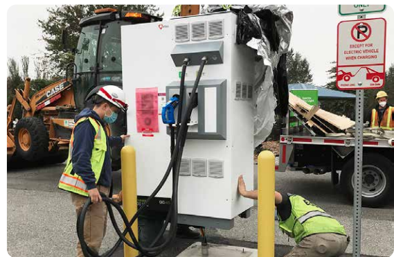
Installation of a City Light EV fast charger.
