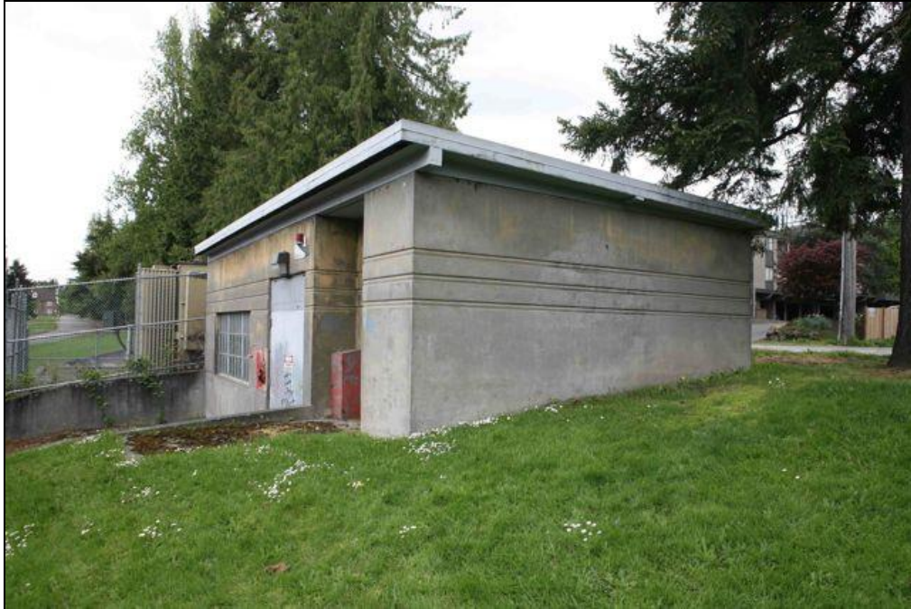
Photo of Building 42 by Artifacts Consulting, Inc., 2009.
