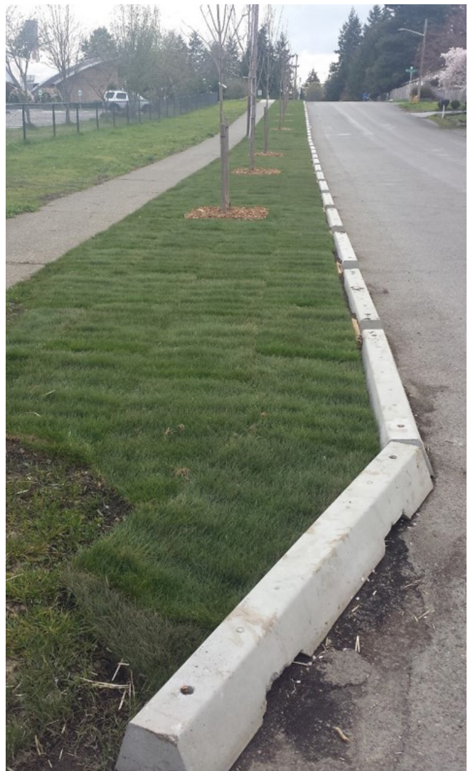
Example of a low-cost sidewalk.
