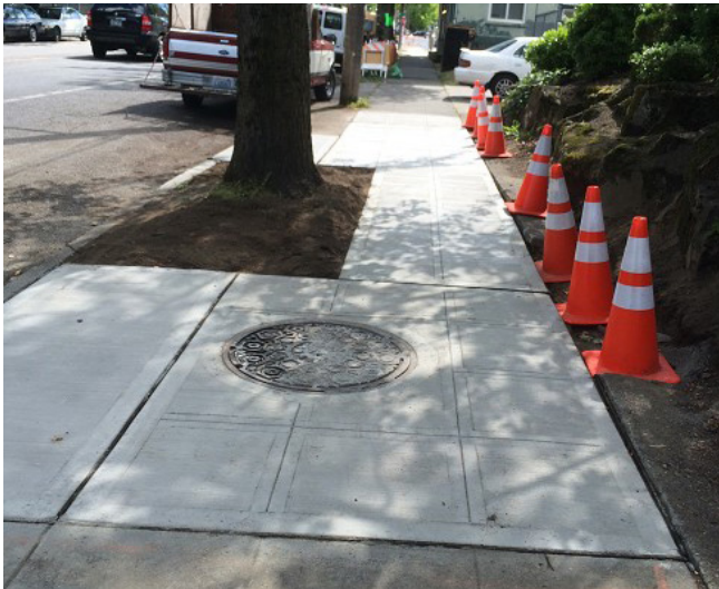
Concrete sidewalk repair on E Cherry.
