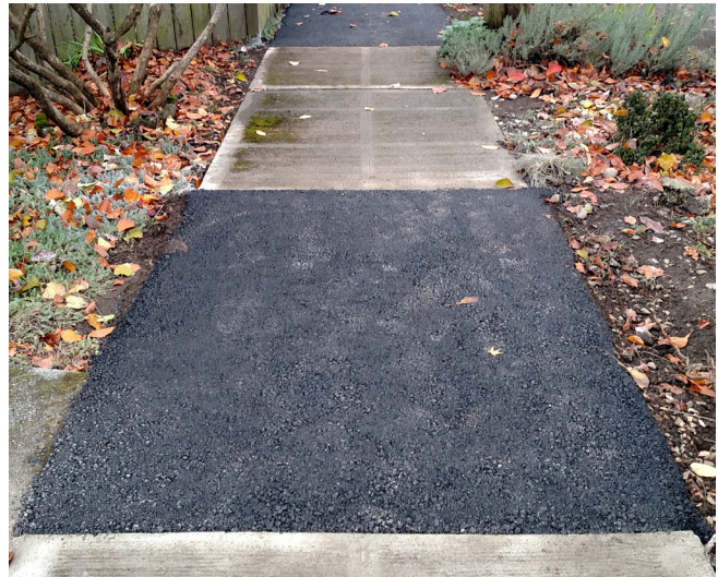
Asphalt sidewalk repair on Charles St
