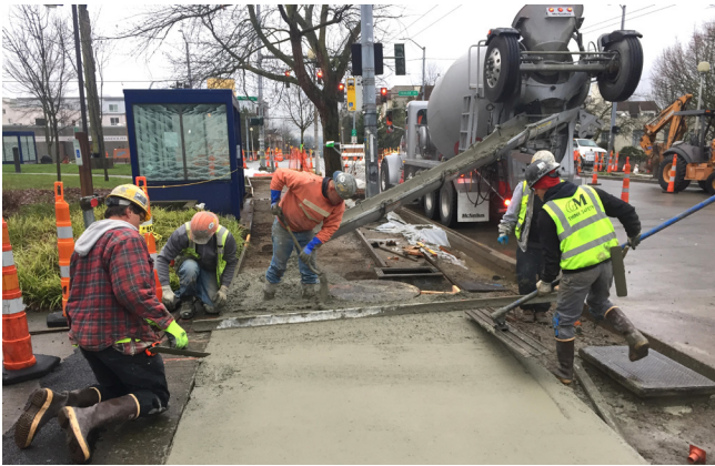
23rd Ave corridor improvements project.
