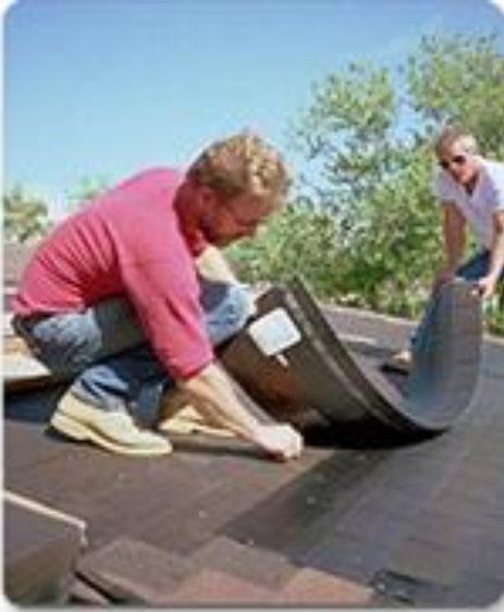
Installing solar shingles
