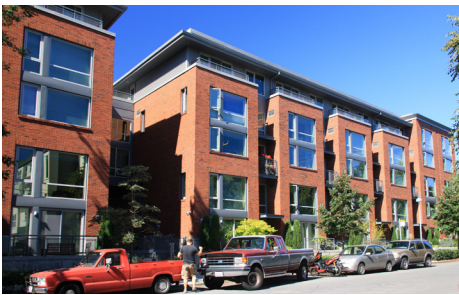
Vertically articulated bays break down the facade scale.
