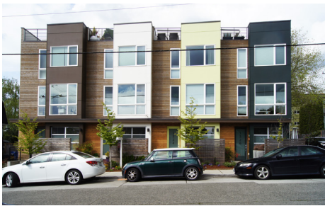
Awnings, façade rhythm, modern bay windows, and a finer grain material texture provide human scale detailing.
