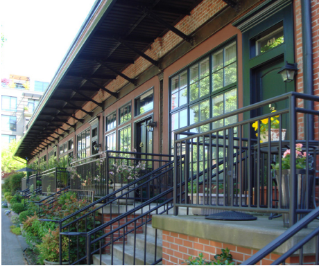
Raised entries that create a private stoop at residential entrances, with high transparency railings that facilitate street interaction.
