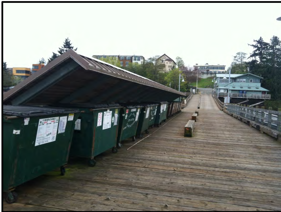
Figure 1. Covered Outdoor Storage of Solid Wastes.
