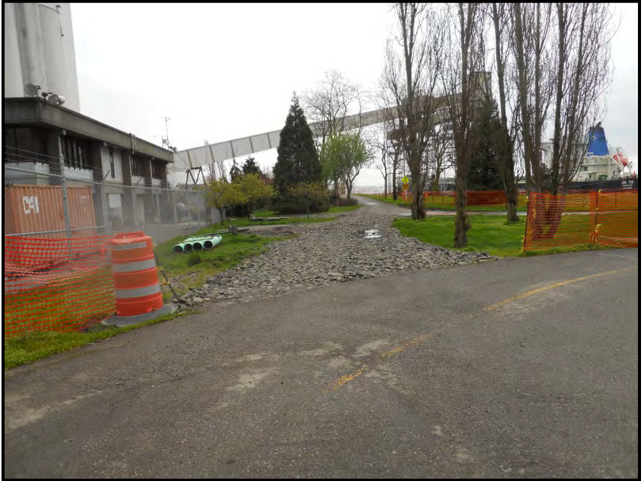
Figure 7. Stabilized Construction Entrance Access .
