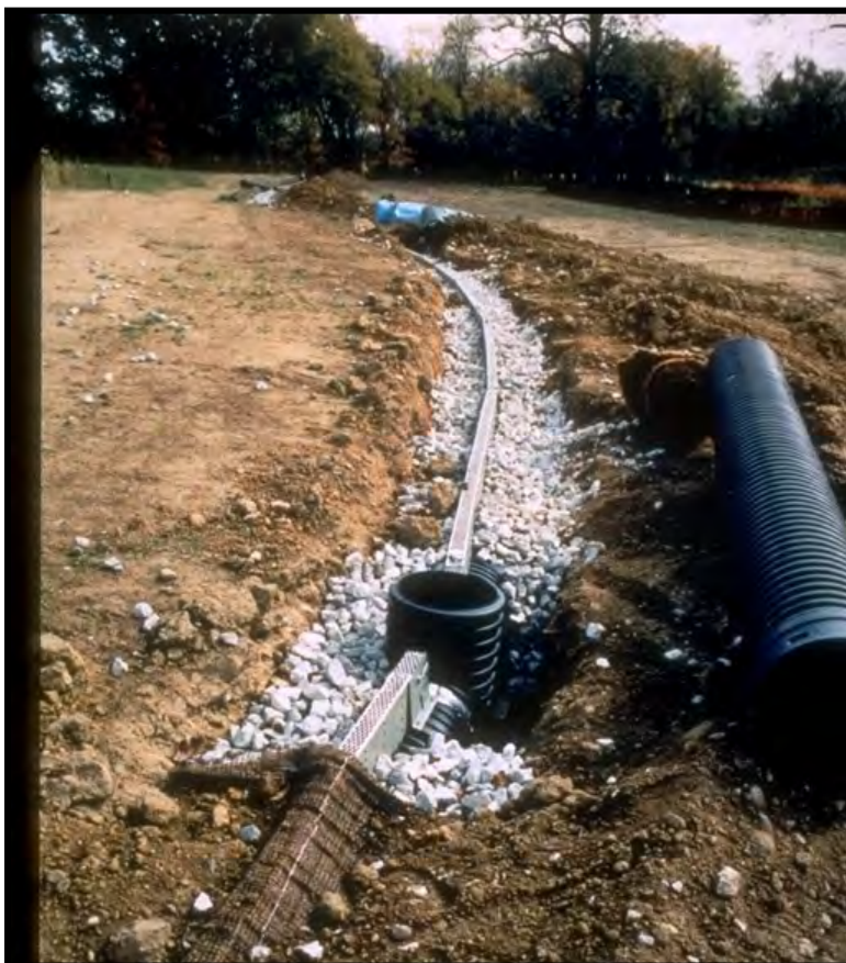
Figure E.7 E.6 . Level Spreader Prior to Backfill and Downstream Stabilization.
