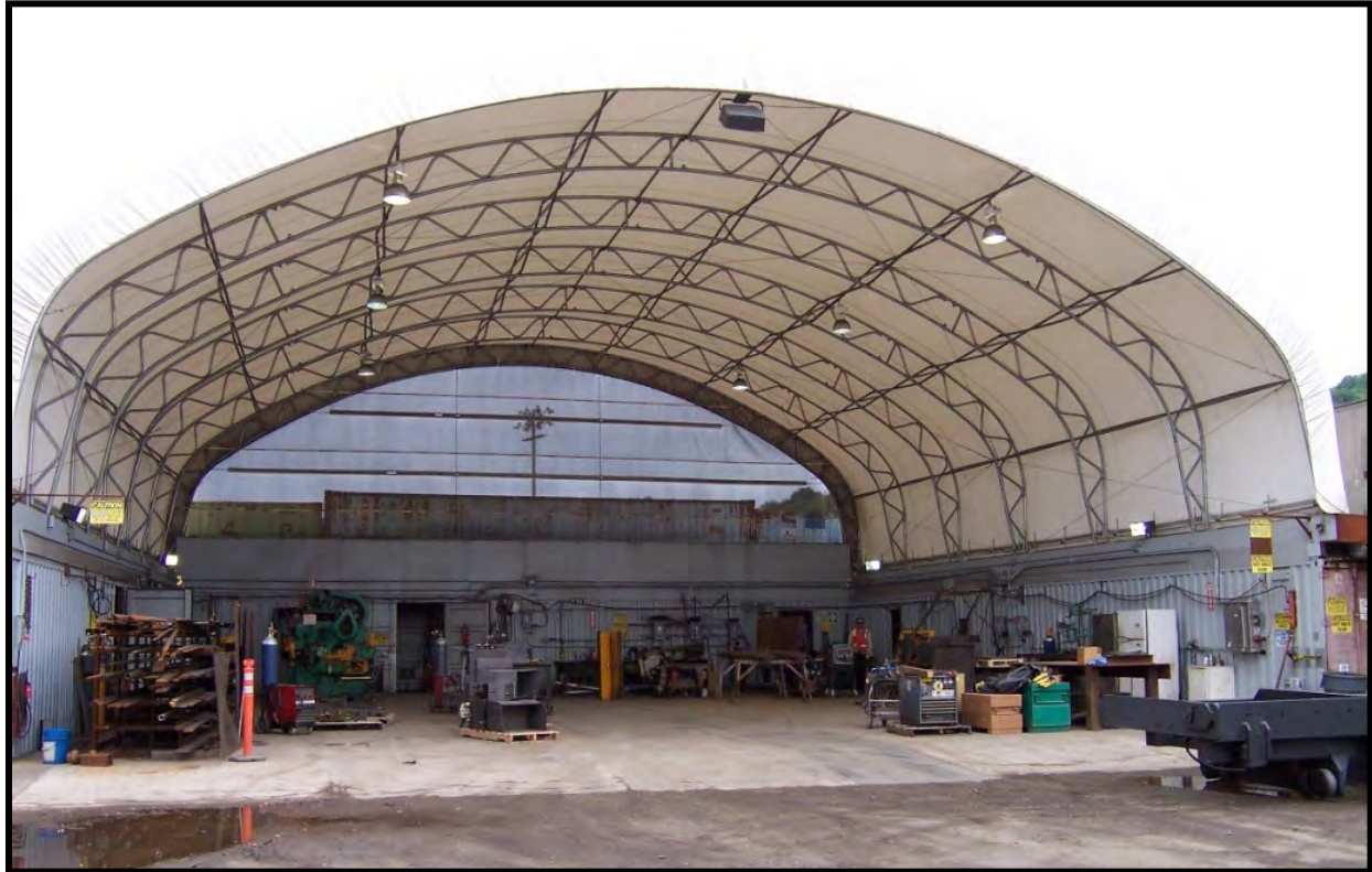
Figure 10. Structure Used To Cover Manufacturing Activities.
