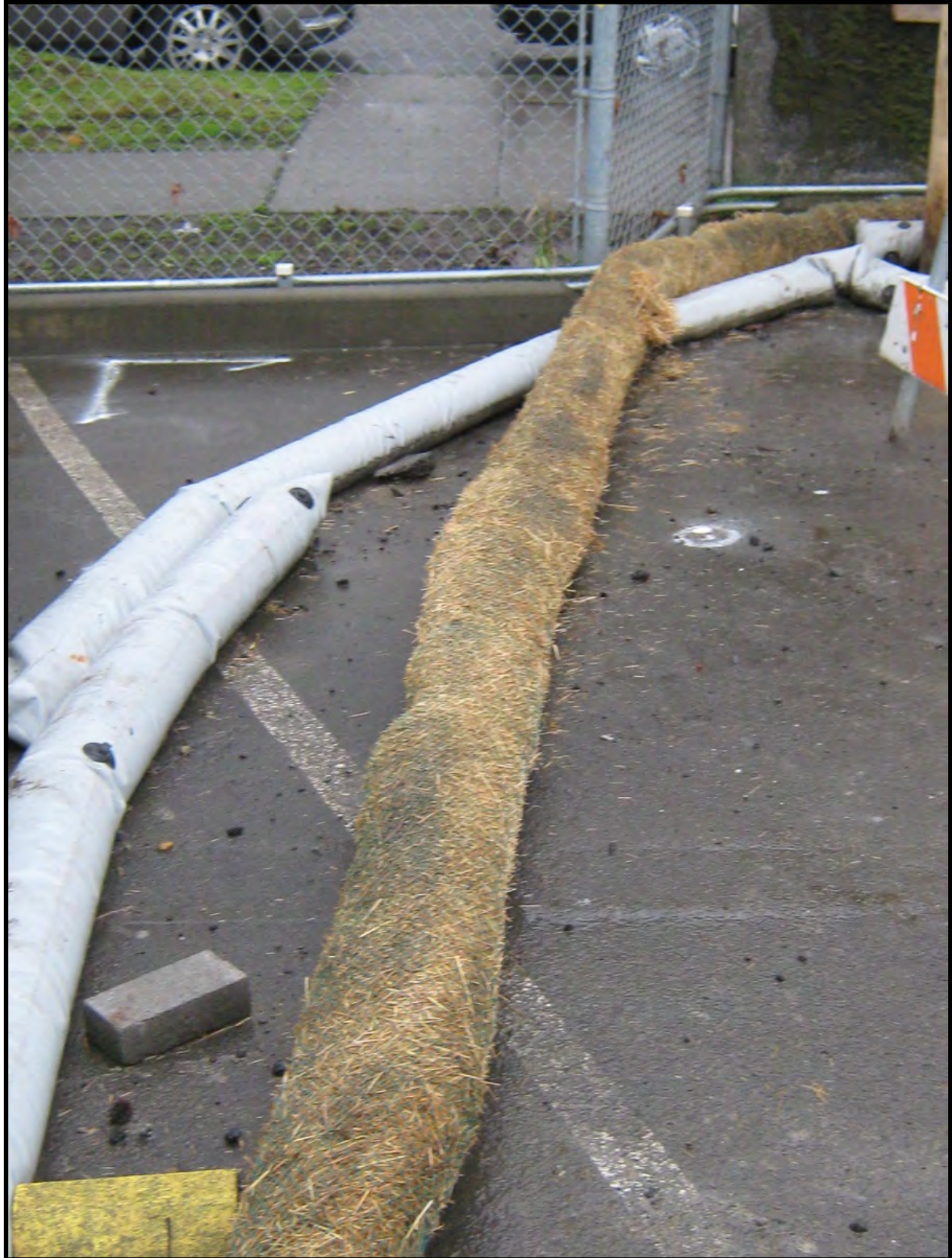
Figure 16. Curb and Gutter Barrier.
