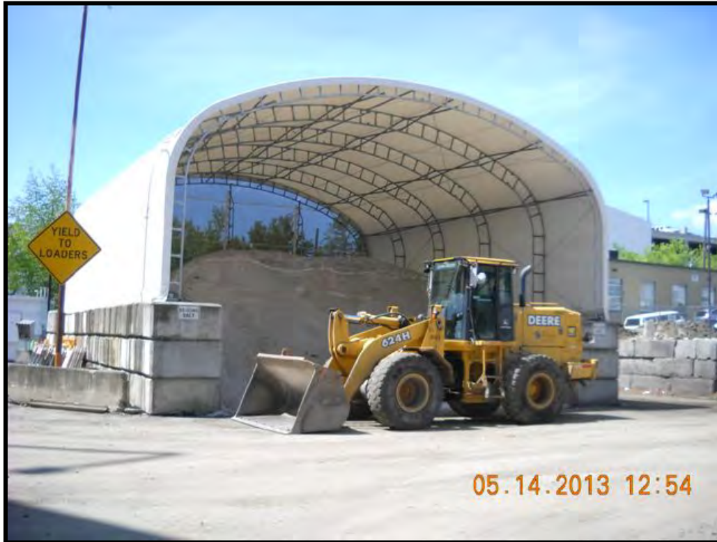
Figure 12. Covered Storage Area for Erodible Material (gravel).
