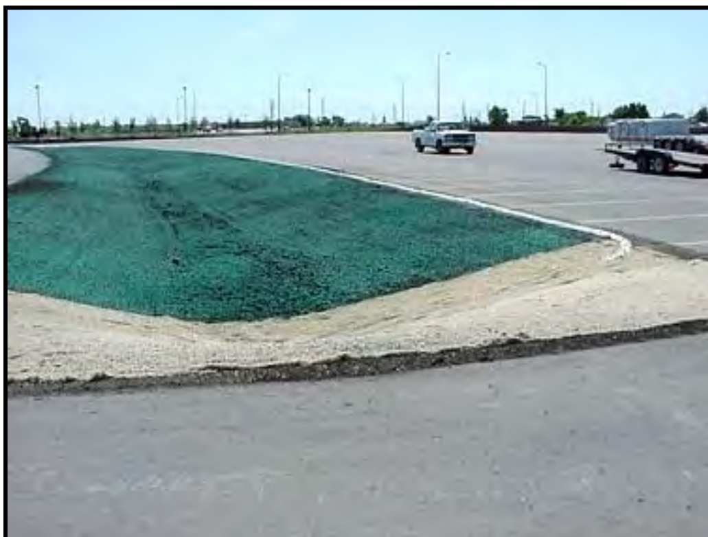
Figure 1. Hydroseeding Method.
