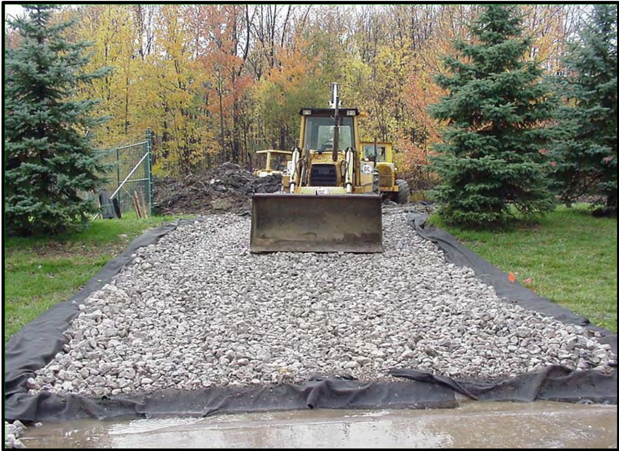
Figure 6. Stabilized Construction Entrance Access .
