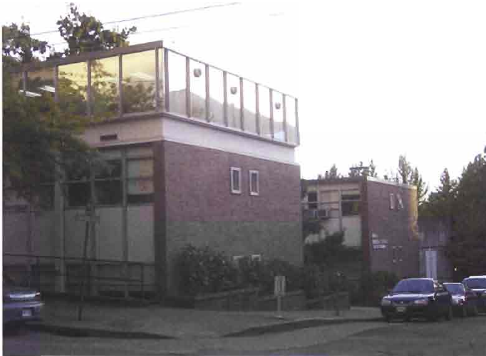
Above, oblique view looking southwest at the primary east and north facades, with the East Wing at its third story addition in the foreground, and the West Wing in the background.
