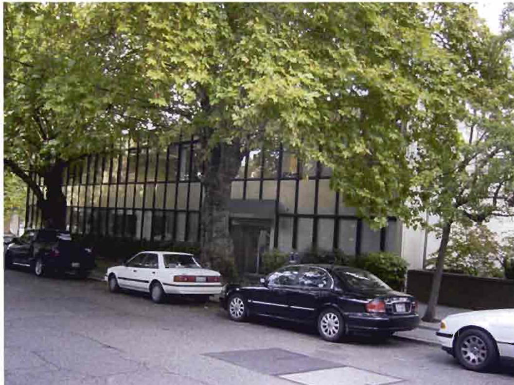
Above, an oblique view of the west facade on Boylston Street.
