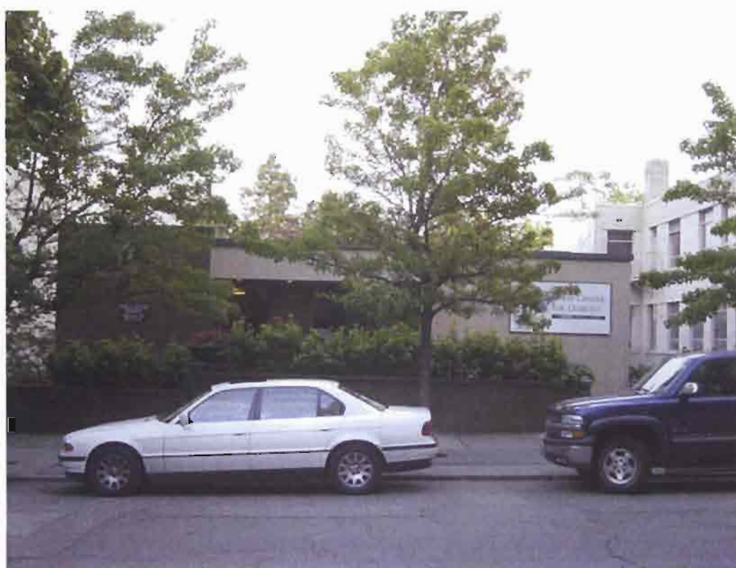
Below, view of the primary west facade and entry off Boylston Avenue.
