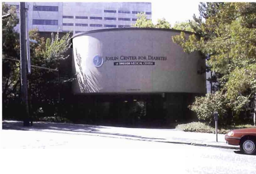
Above, view of the vehicle entry off Broadway (east facade).
