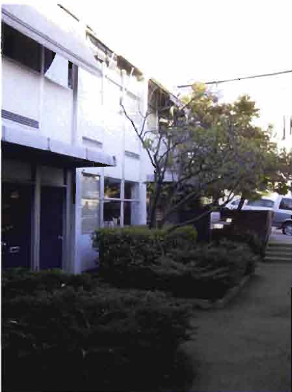
Below, detail view of the west wall in courtyard.
