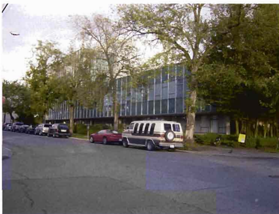
Above, view of the building's original western section, north and partial west facades.
