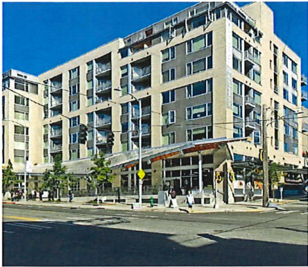
This building is a positive example of a six-story mixed-use building that is a good fit for both the Character Core and General Commercial Character Districts.
