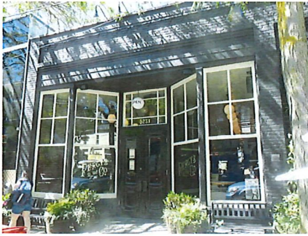
Historic Ballard Ave. NW storefronts engage with the public sidewalk and street.
