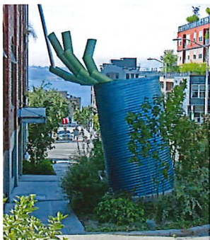
The Buster Simpson designed cistern in Belltown adds a whimsical and functional stormwater detention.
