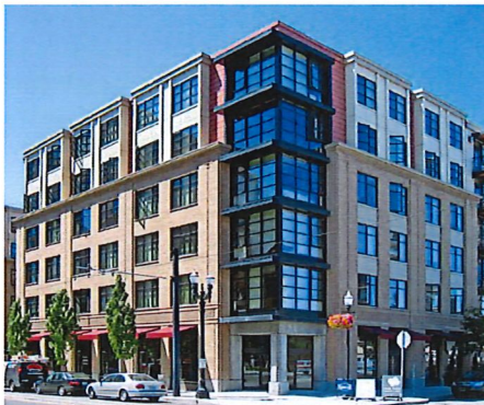
The vertical and horizontal banding is expressed differently in the lower and upper portions of this building, providing a unifying theme while reducing the perceived bulk.
