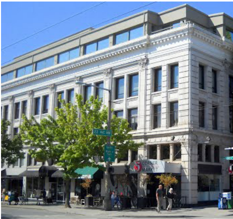
This strong facade composition, detailing, and high-quality materials establish a clear commercial character.
