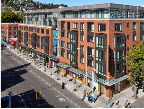
This building's design, details, and quality materials would fit well in Ballard. The upper floors are clearly residential.
