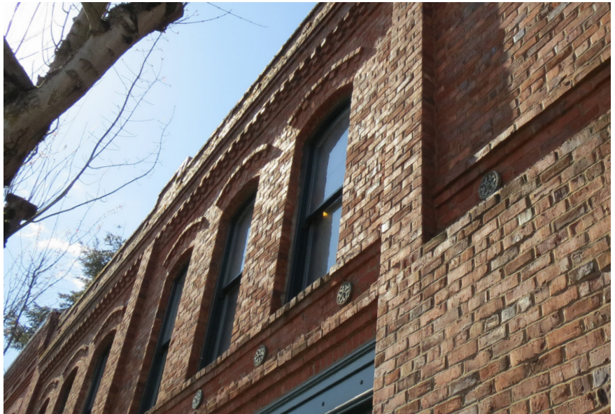
Scale and texture can be achieved when using one material as shown in this brick building that incorporates details like continuous sills, segmental brick arch, and a cornice with a dentil band.
