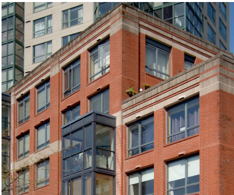
Changing height at the corner of this development reduces the bulk.
