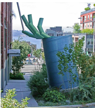
The Buster Simpson designed cistern in Belltown adds a whimsical and functional stormwater detention.
