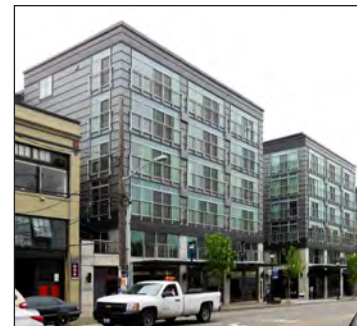
The modulation or division of this building into two sections with a recessed middle portion helps to keep it in scale with the neighborhood.
