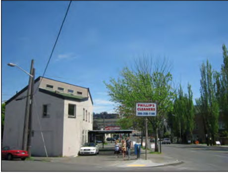
In areas lacking well-defined character, new development should extend established Pike/Pine neighborhood character.
