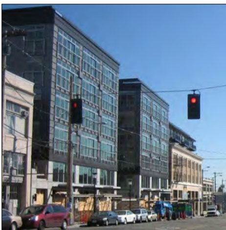
Through the use of setbacks, courtyards or other interruptions in the street-facing facade, wider structures can relate better to established scale conditions.
