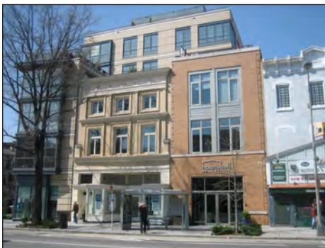
In this successful example, structures to the left, right, and above the center structure are additions.
