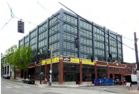
A successful example of an addition that was set back less than 15'. The contrast between the character structure and the new addition was achieved through materials, subdued colors, simple fenestration and changing the original vertical grid orientation to a horizontal emphasis.
