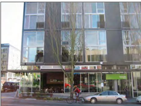
Use of modern materials
