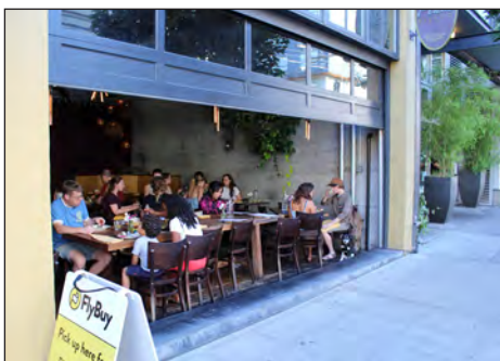
Design and use of ground floor space to encourage interaction between new development and the public street environment.
