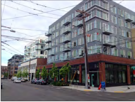
Large development site with massing that creates the appearance of a grouping of smaller structures.
