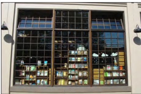
Window trim detailing.
