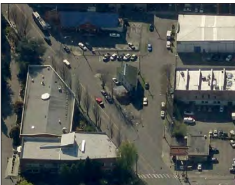
The “bowtie”-style intersection is shown at the intersection of Madison Street and Seneca Street.
