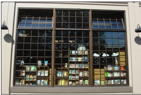
Window trim detailing.
