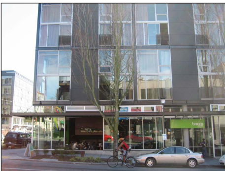
Use of modern materials
