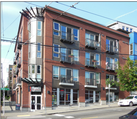
This building façade does not feature storefront entrances at different levels and so is perceived as one continuous façade that does not respond to the topography.
