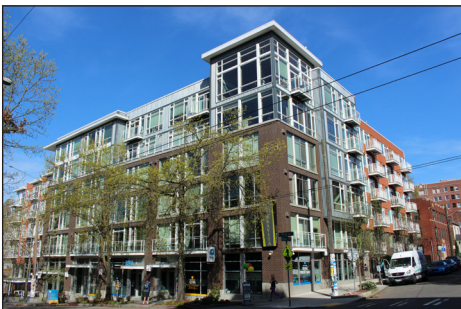
The storefronts on different levels accentuate the differences between the two building façades and appear to “step up” with the topography.
