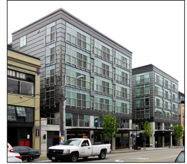
The modulation or division of this building into two sections with a recessed middle portion helps to keep it in scale with the neighborhood.
