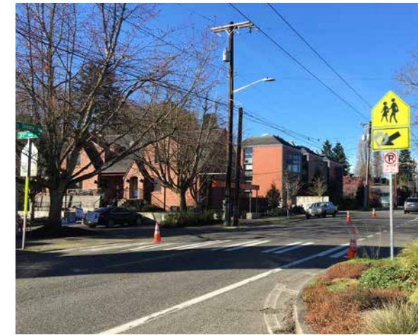
Crosswalk and signage on E Denny Way
