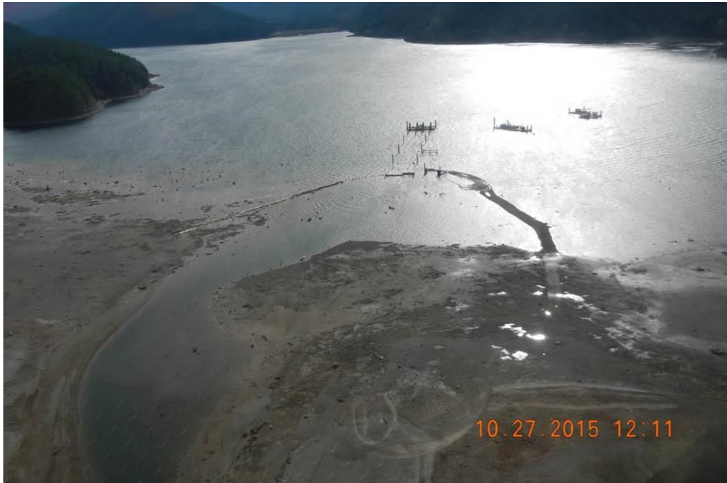
MLTPP – PP2 – PP1 (L to R); Discharge Dike (middle); Outlet Channel (left bottom)
