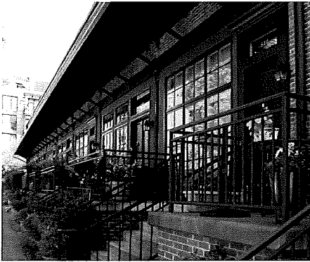
Raised entries that create a private stoop at residential entrances, with high transparency railings that facilitate street interaction.
