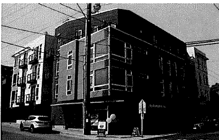
Articulated building massing both horizontally and vertically breaks down the building's scale.
