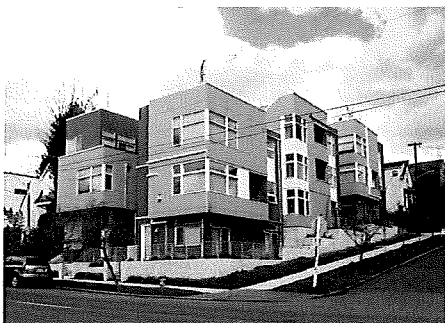
Broken-up building massing avoids a monolithic form.
