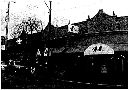
Commercial facades exhibiting historic character provide a model for future street level uses.
